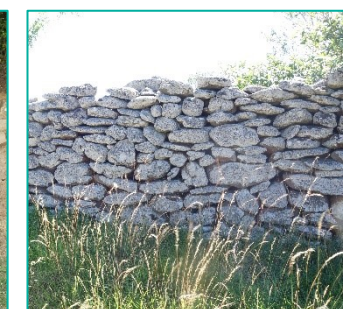
Mur, Chalagnac, Bonnac
